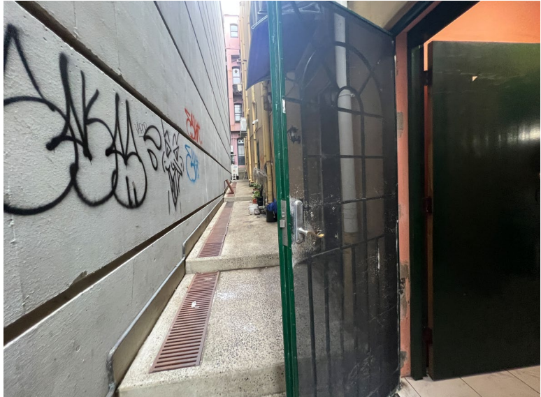
rear access to site from Kent St
